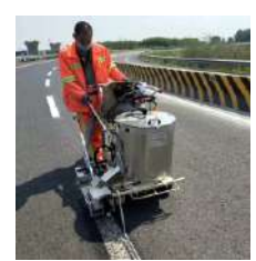
Thermoplastic Road Marking
